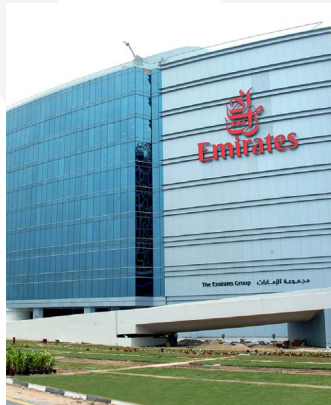
Emirates Airlines Headquarters - Dubai
