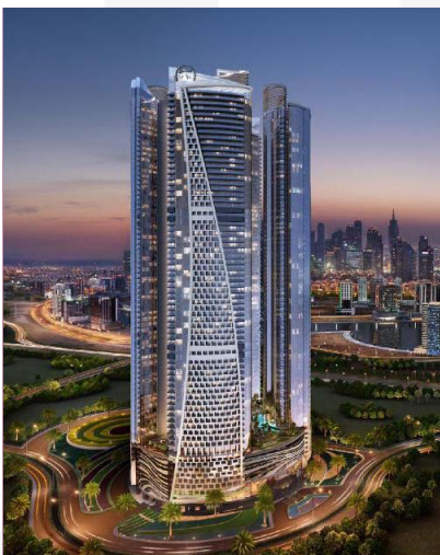
Paramount Towers Damac - Dubai
