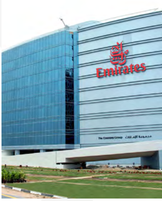
Emirates Airlines Headquarters - Dubai
